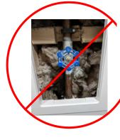
Cannot see where pipe comes through - try to pull back insulation and use phone camera to view pipe at breakthrough.
