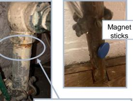
Galvanized pipes have "threads" at connections.
