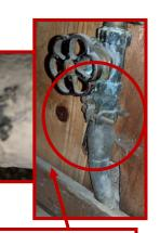
Lead pipes **widen** at base and often form a "**bulb**."
